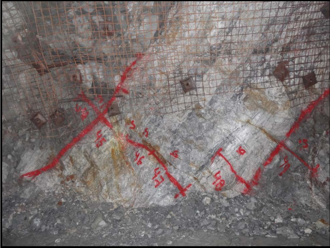
Early exposure of the Inca 1 vein in the Casposo underground. 2380NW - CHIN_00001: 2.20m at 18.47g/t gold and 1380g/t silver or 41.48g/t Au_Eq from 0.50m Incl: 0.60m at 49.53g/t gold and 4145g/t silver or 118.61g/t Au_Eq from 2.10m
